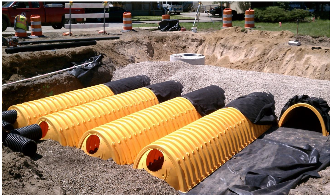
Figure 4.5: Underground Storage Main Features [14]
